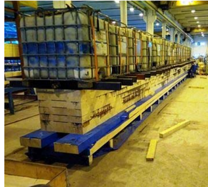
Block gluing of columns
