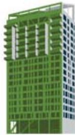
Mjøstårnet Norway 18 Stories Under Construction
