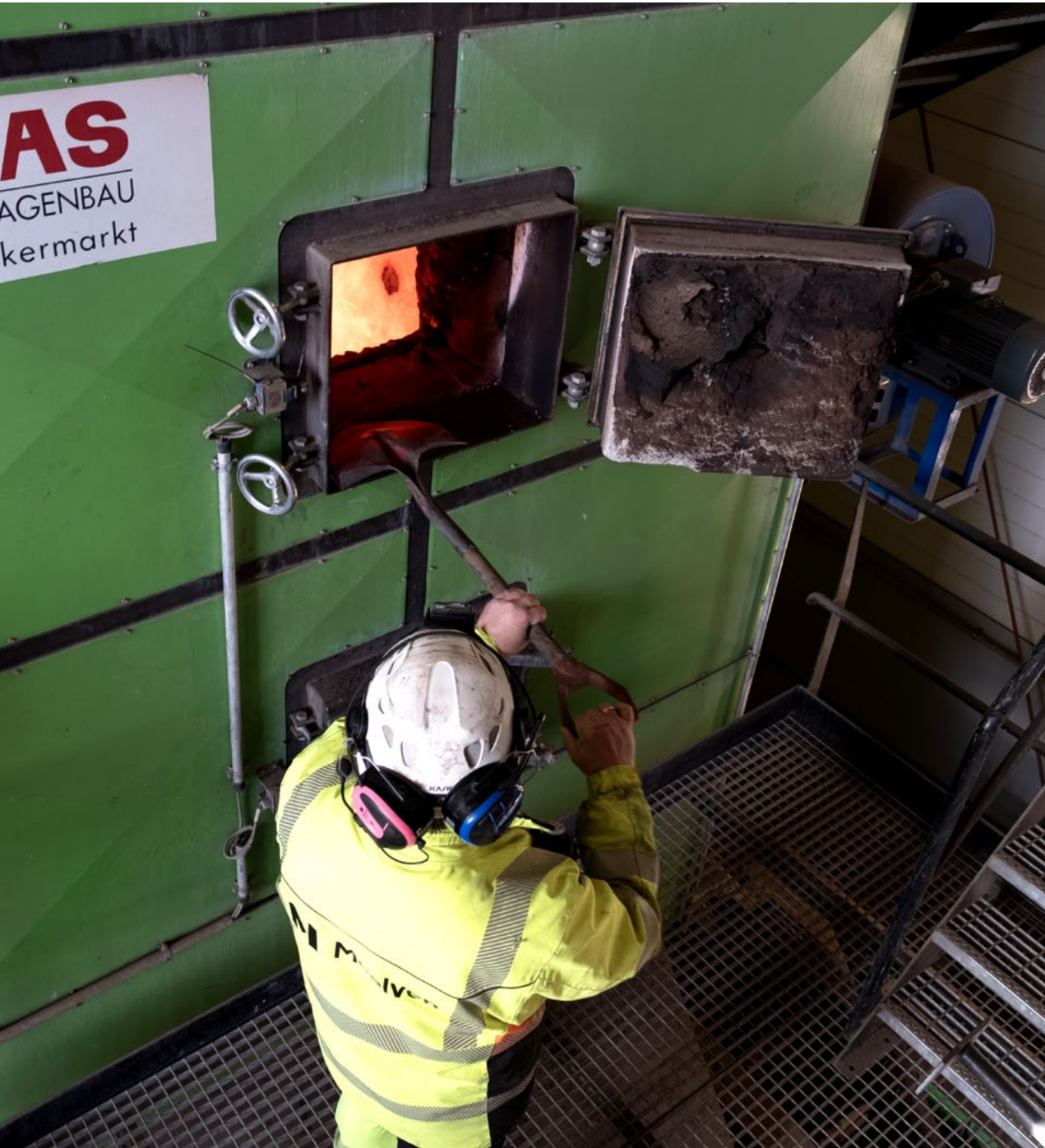
Visual control of the combustion process. The temperature inside the combustion chamber can reach up to 1000 degrees C.
