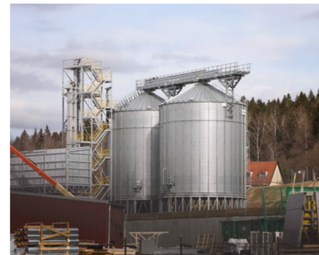
Storage silos for wood pellets at Moelven Pellets AB in Karlskoga. Not all residual raw material is used for our own bioenergy production. In both Norway and Sweden, Moelven has plants that process residual raw material from the wood industry into pellets for external sales.
