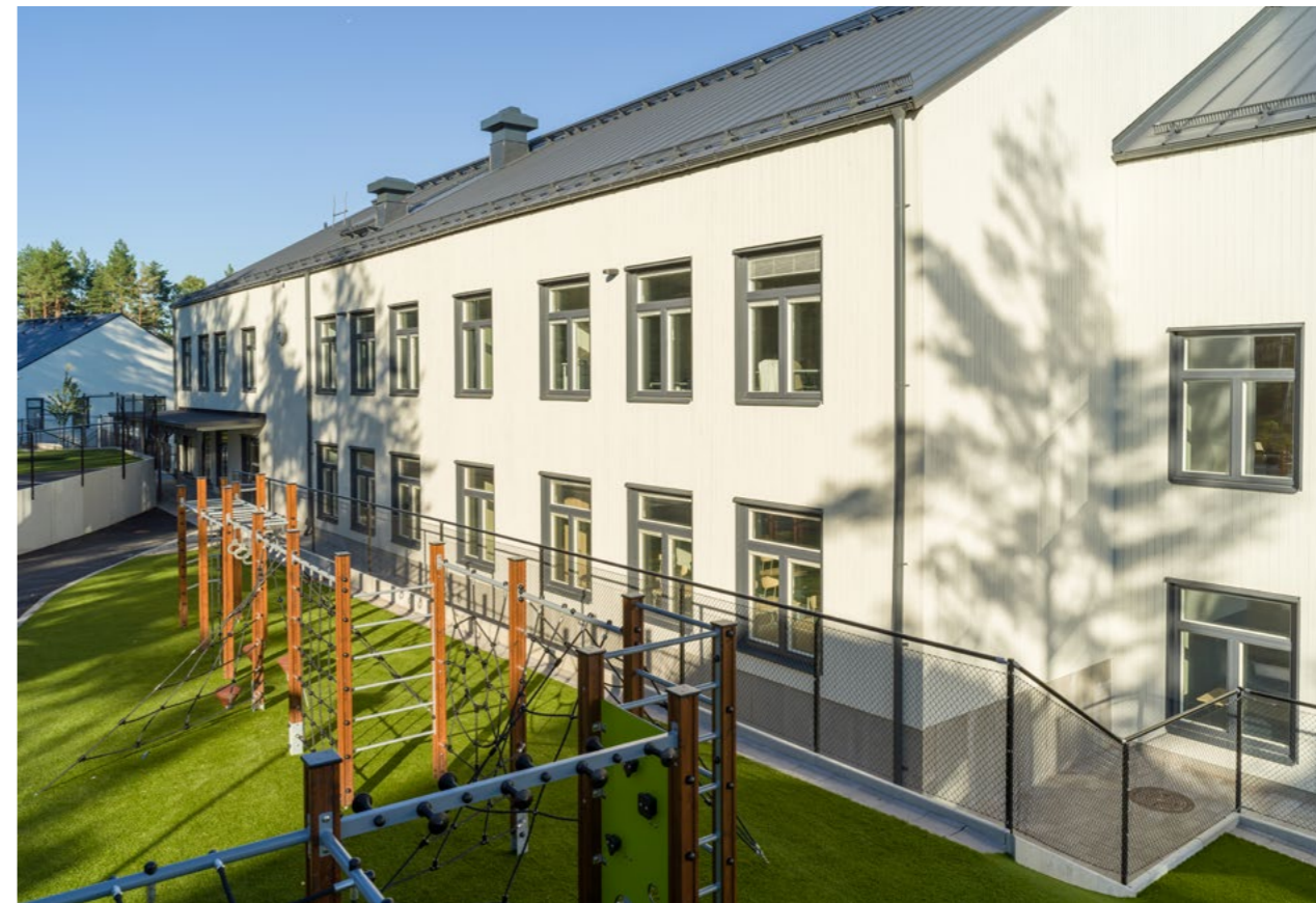
Bro Målarstrand in Upplands-Bro has a new environmentally certified school building (Nordic Swan Ecolabelling) with an associated sports hall, completed in just one year by Moelven Byggmodul AB. Photo: Andreas Hyllthén
