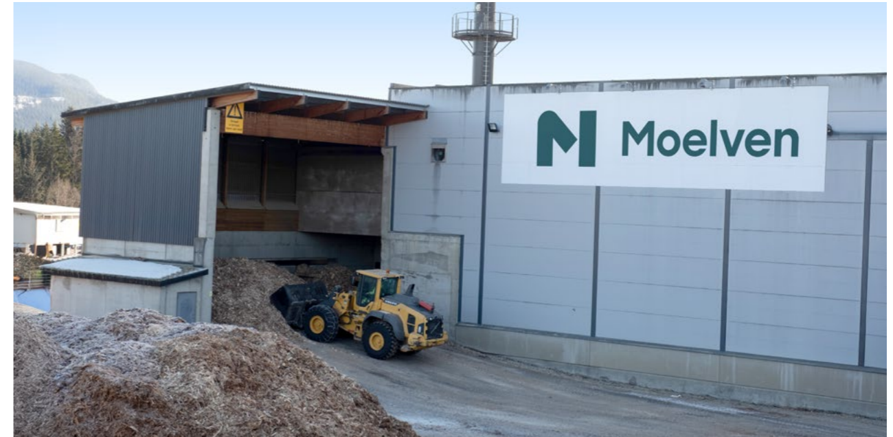
Loading of biomass at Moelven Mjøsbuket AS. The biomass mainly consists of the bark from the sawn timber, mixed with other wood chips to achieve the desired moisture content for the combustion process.
