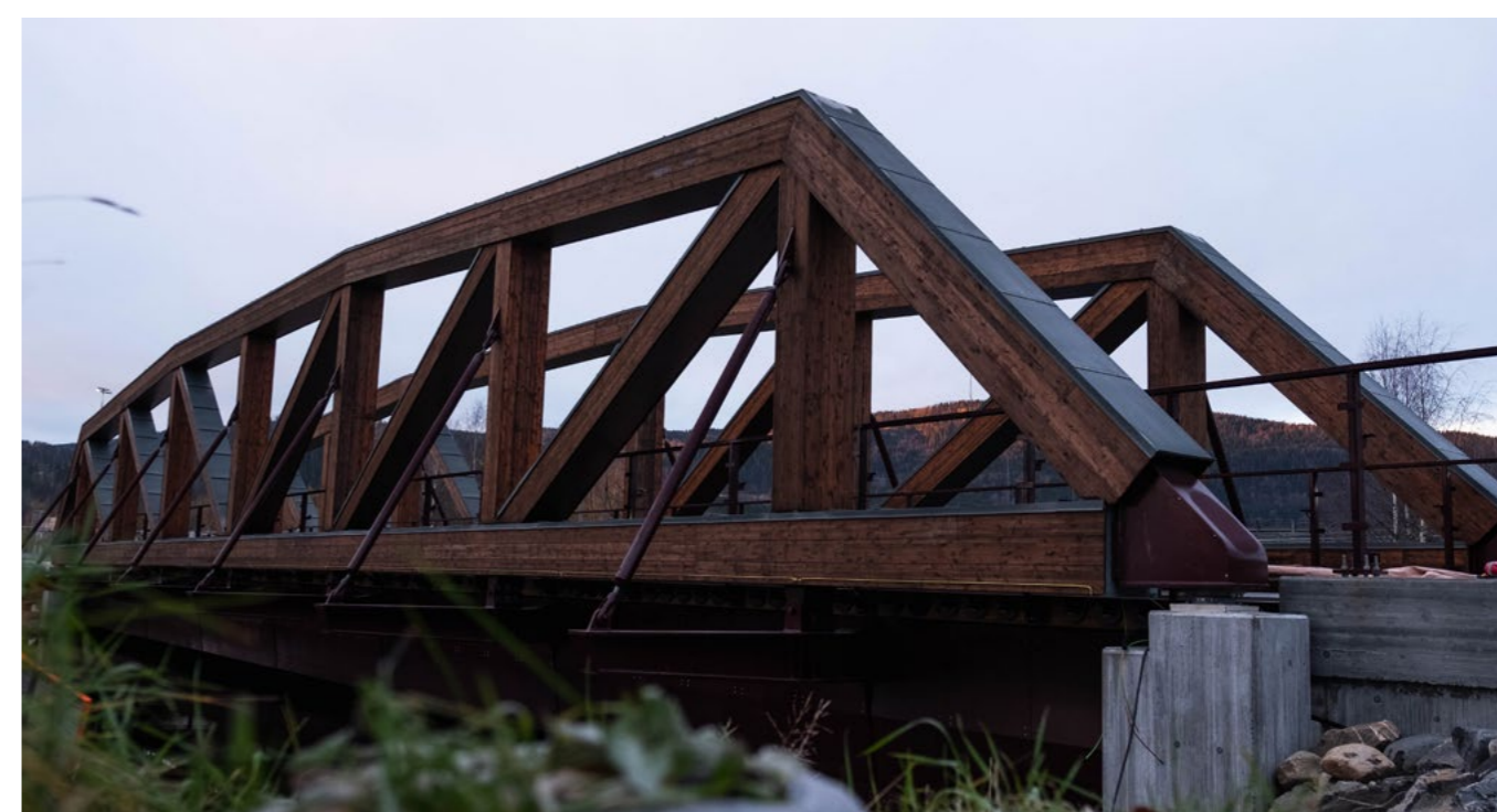
Lillehammer municipality has built a brand new truss bridge for pedestrians and cyclists in glulam from Moelven in 2024.
