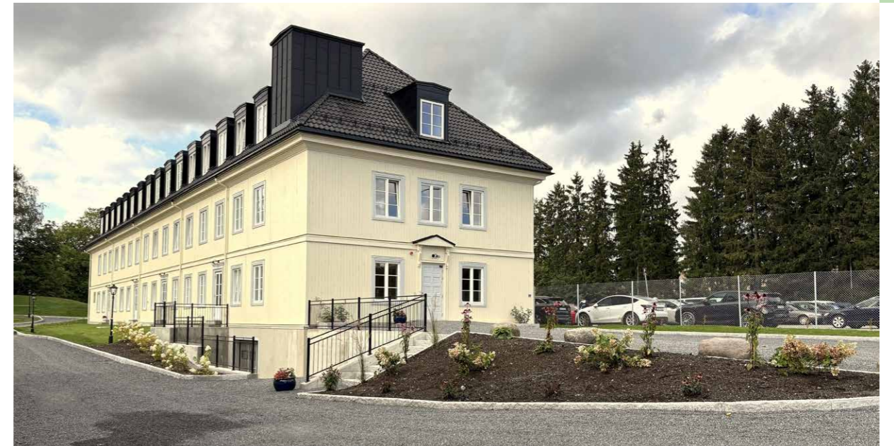
Blindern Studentehjem, produced by Moelven Byggmodul AS with Heftig cladding provided by Moelven Spesialtre AS.
