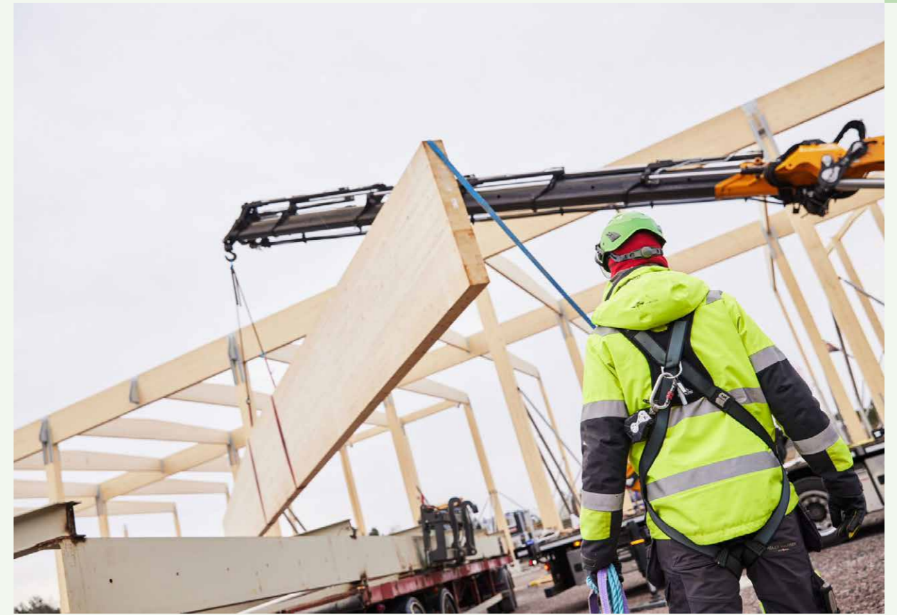
Precise and safe handling of glulam structures during installation.
