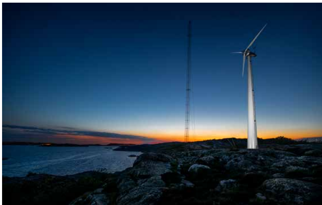
The first prototype of a glulam wind tower was installed on Björkö in the Gothenburg archipelago in the spring of 2020.
