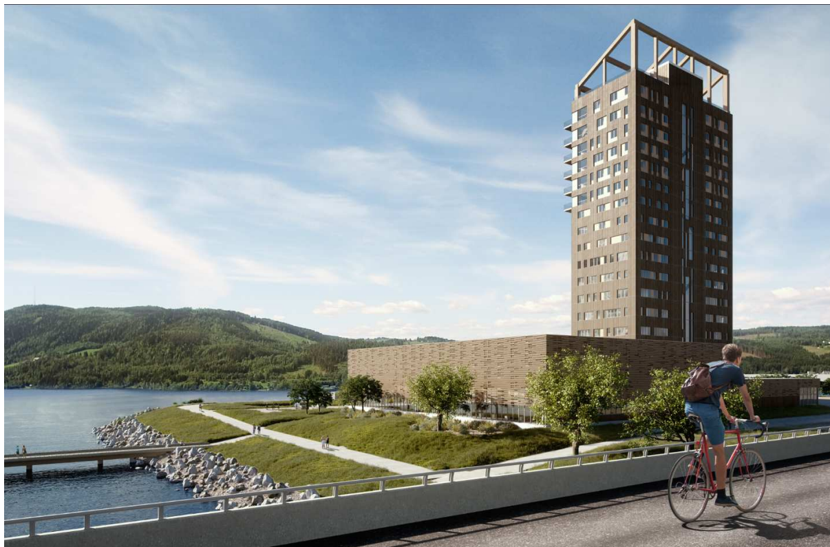
«Mjøstårnet» - The world's tallest wood building, scheduled for completion in 2019. Moelven Limtre AS will supply and assemble all wood structures in the period from September 2017 to April 2018.
