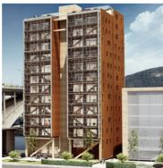
Construction of the world's tallest wood building, "Treet" in Bergen, started in the fourth quarter of 2014. The building will, when completed in the autumn of 2015, consist of 14 storeys and be 51 metres tall. The load bearing glulam structures will be supplied and installed by Moelven Limtre AS.
