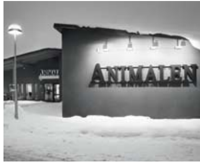
The small animal clinic, Animalen, in Södertälje, Sweden, was recently erected using building modules from Moelven.
