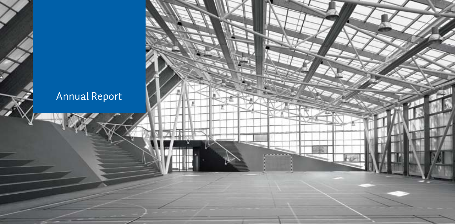
Glulam beams and Finnforest Kerto supplied by Moelven set their mark on the sports and cultural centre, Prismen, at Amager in Copenhagen. The transparent roof provides excellent lighting conditions during the day, and at night the building resembles a sparkling crystal.
