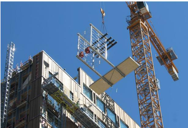
*Figure 17: Hoisting of balconies with tower crane.*
