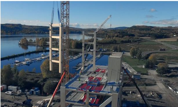
*Figure 16: Hoisting of frames.*
